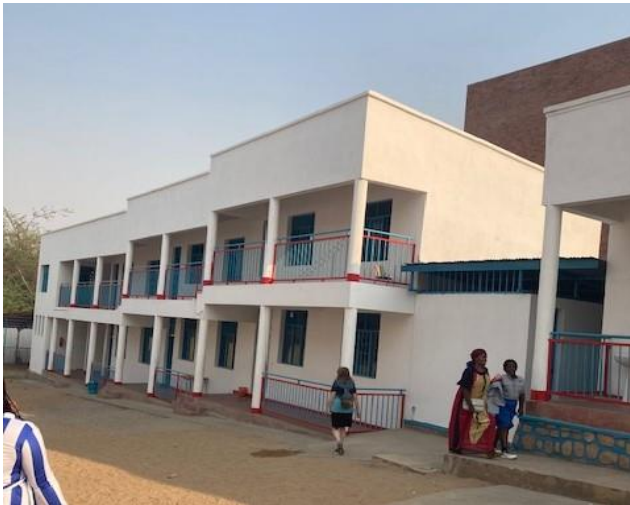
3 New Classrooms- second floor addition
