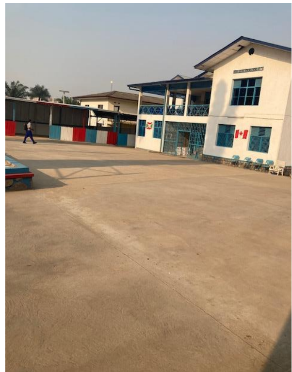
Repaired and paved tarmac of BES, the former Nigerian Embassy, situated on high ground on Avenue du Large.
